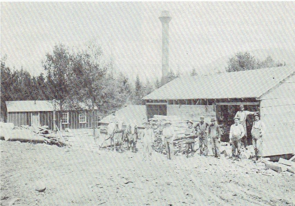
Charles Silver's Birch Mill—1903. On left after crossing the line bridge from Labrador Pond.
