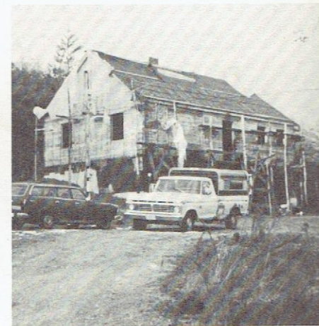
Cellar of Paul & Pat Berube. Near where buildings of Vernal Kimball were.
