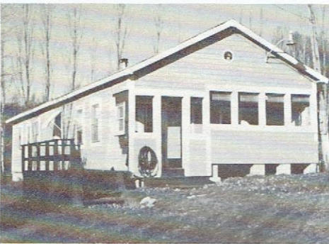
Bill Bryant—Built on the site of the old Blacksmith shop. 1791—Benjamin French. Newton Records had a Blacksmith Shop on the East side of road.
