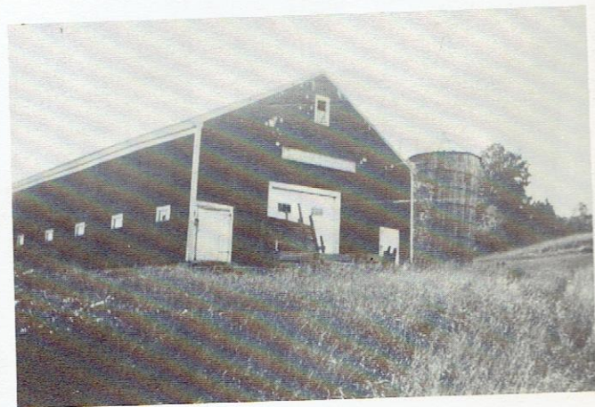
Mose Young barn and silo
