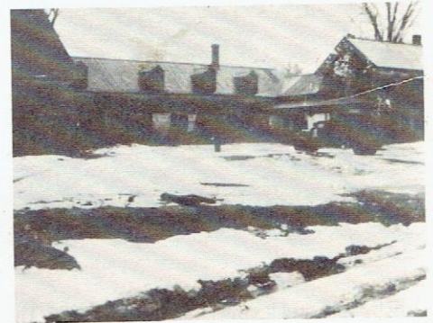
Buildings previously owned by "Bun" Gammon.
