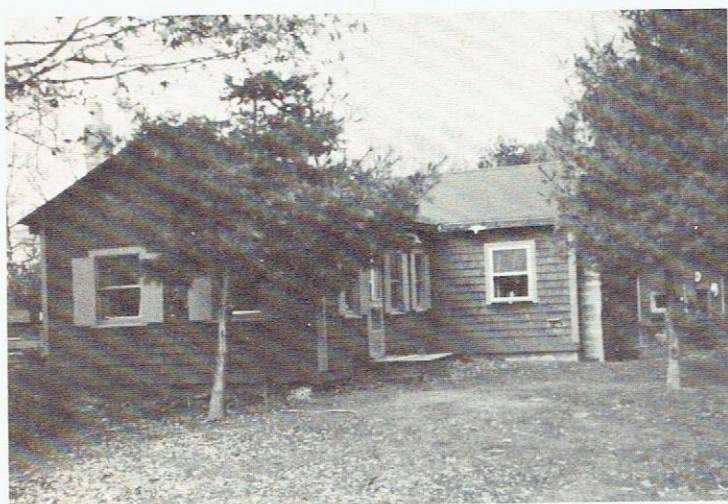
New house of George Bitner. 1858 & 1880 S. Ames—Old buildings gone.
