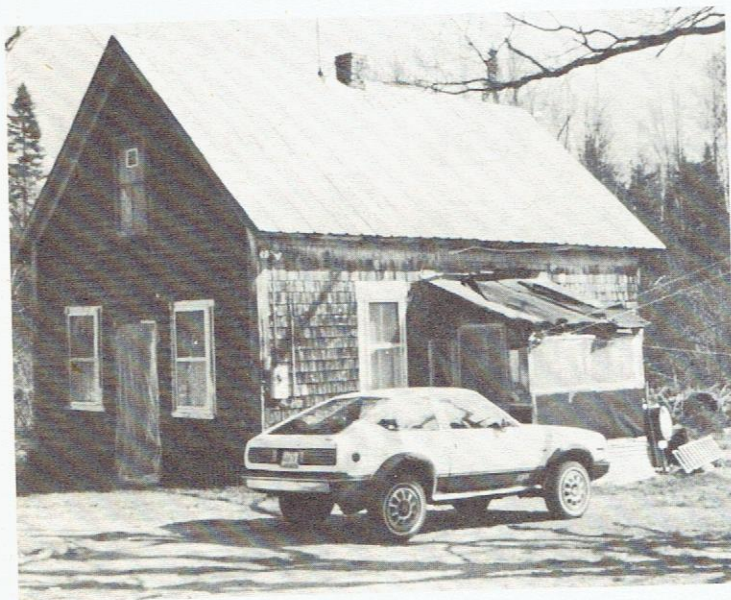
This house was built by John Oldham and John Widber. Vera Gurney now lives here.
